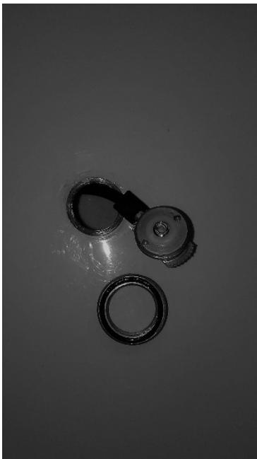
Drill a 3/4" hole in the center of the roof
